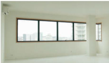
Slimcase is a concept applied to a minimalist view window system, dominated by the glazing look and outwardly appearing to have a structural bonding. The exterior shows a frame with a black silk-screen printed glazing with a fine expression of aluminum.
